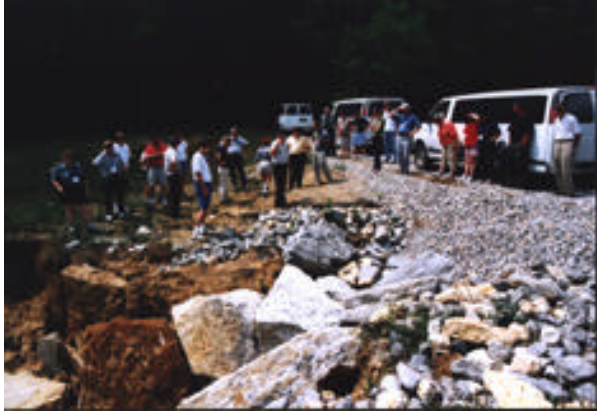
Refuge Specialist Dr. Joe Robb , center, explains the severe washout that occurred at the spillway of Old Timbers Lake with the torrential rains our region experienced this past spring.
